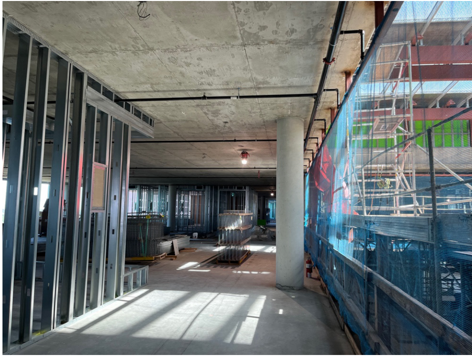
Office level 7 -framing
