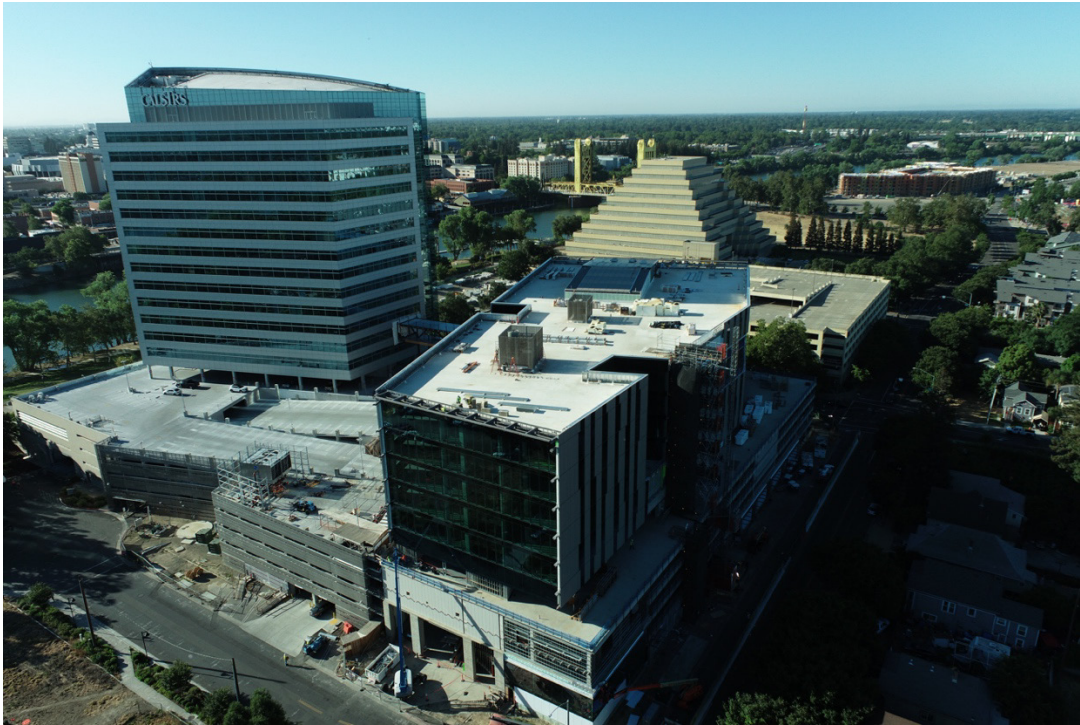
Northwest side of building
