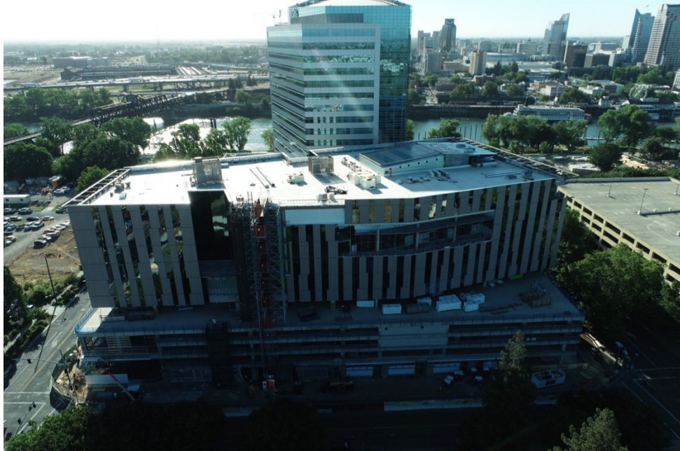
West side of building
